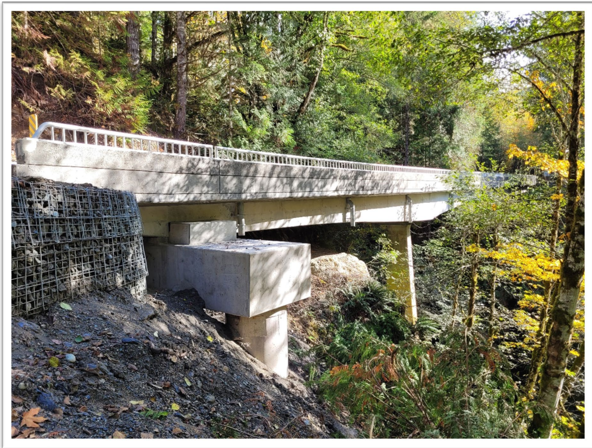
“Upper Finney Creek Bridge”
