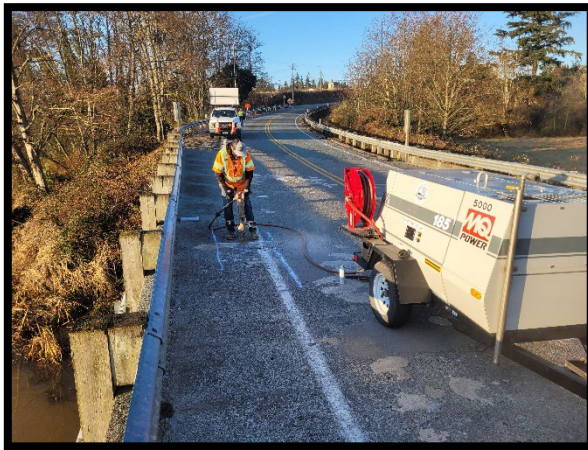
Bay View-Edison at Joe Leary Slough Bridge – jackhammer used to expose rebar for measuring and spacing, some of the information that went into the deck rehab project.
