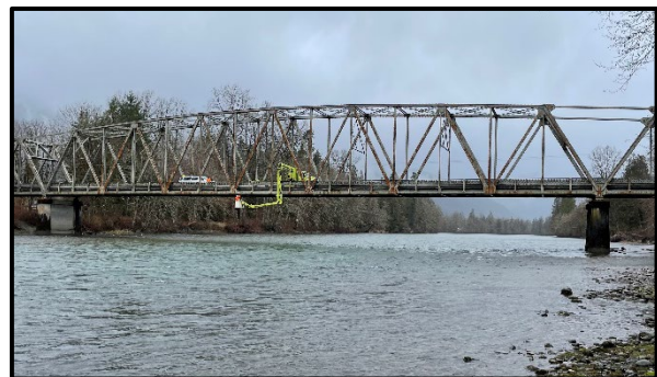
Skagit River Marblemount Bridge, UBIT inspection
