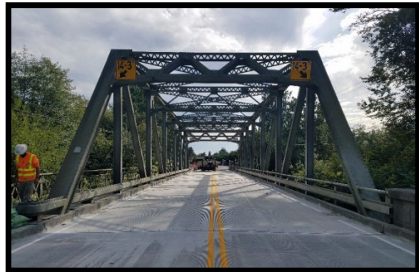
Samish River Bridge - Vertical Clearance Signage
