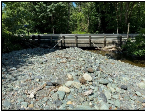
Mill Creek channel upstream of bridge.
