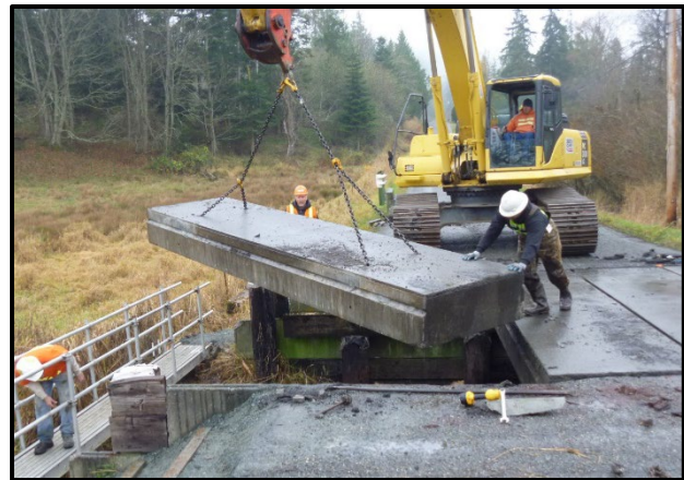
Campbell Lake Outlet receiving new timber cap, 2013
