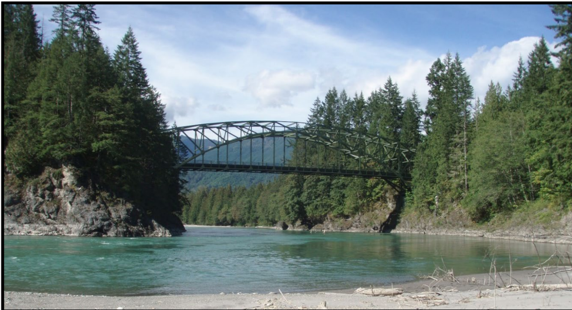
Dalles Bridge near Concrete (Concrete-Sauk Valley Road)
