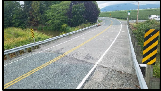
Bay View-Edison at Joe Leary Slough Bridge
