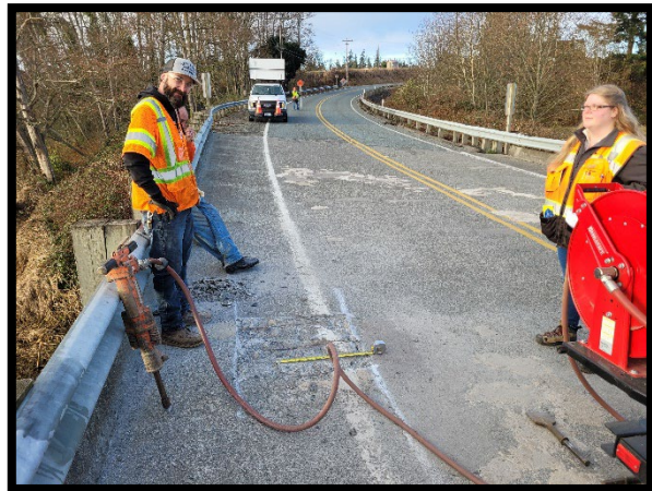
Bay View-Edison at Joe Leary Slough Bridge – jackhammer used to expose rebar for measuring and spacing, some of the information that went into the deck rehab project.
