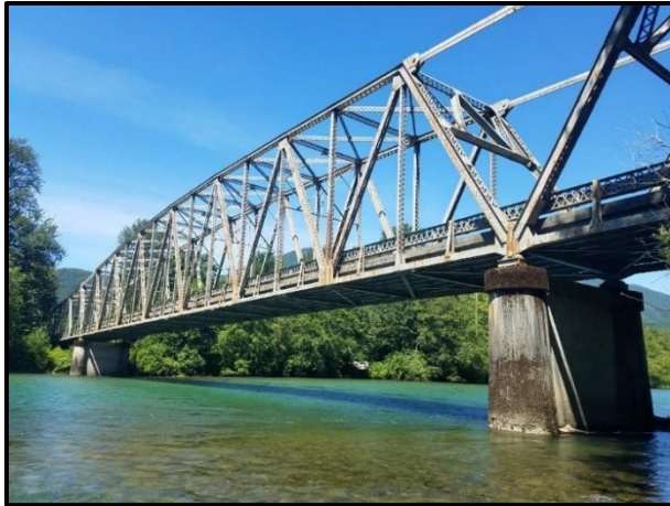
Marblemount Bridge – Skagit River
